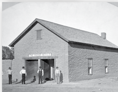
Salt River Herald Building
